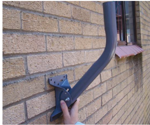
Figure 4-3 – Pole Assembly
