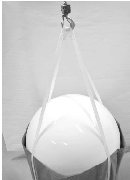
Figure 2-31: ADU installation, 4 lifting straps on crane hook
